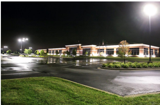
Outdoor car parking lot
